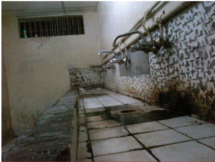
A bathroom from Dry Dock Detention Center
